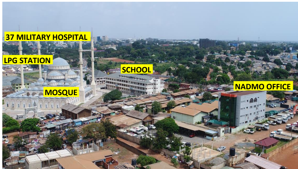
Plate 10 : Multi-storey residential units within the inner LPG hazard zone Source: Fieldwork, 2019
