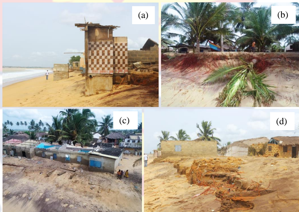
Figure 5.3: The dire state of Anlo Beach: (a) collapsed bathhouse (b) eroded beach face, causing the uprooting of coconut trees (c) some collapsed houses due to storm surges (d) eroded beach face
