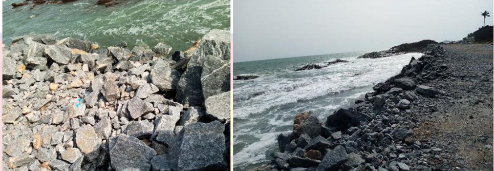
Figure 2.9: Materials used for hard-engineered sea defence structures along the coast of Ghana. Source: Author (2022)
