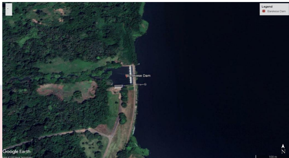
Figure 2.5: The Barekese Dam on a tributary of the Pra River
