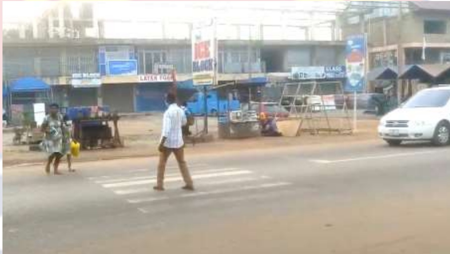
Figure 14: Plate showing a nearly wiped-out zebra crossing
