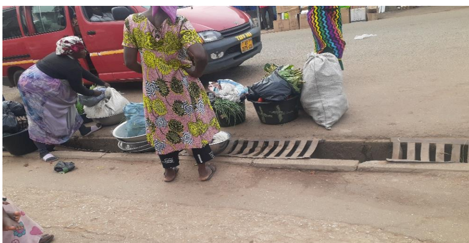
Figure 13: Metal slabs covering gutter caved-in
