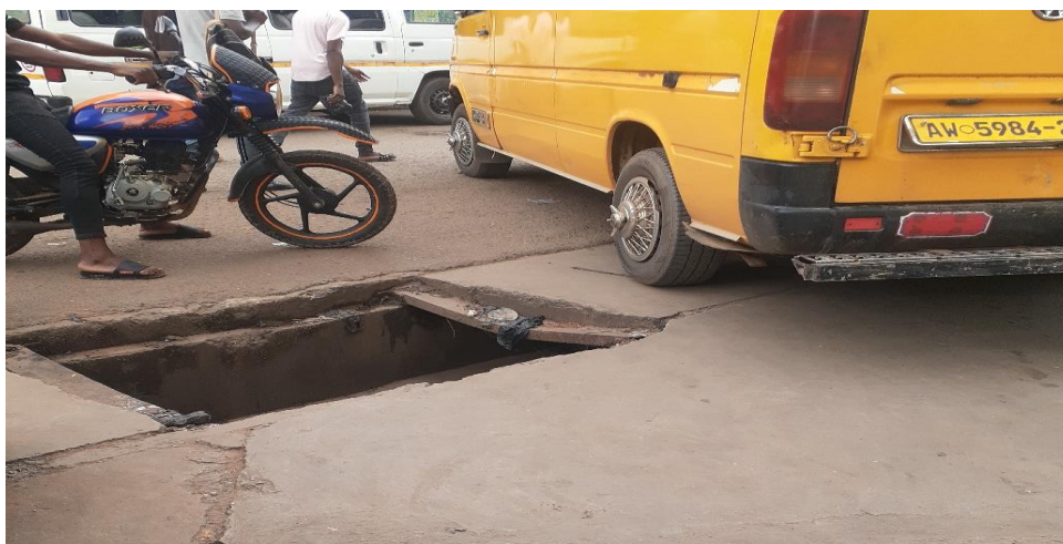
Figure 14: Exposed drainage
