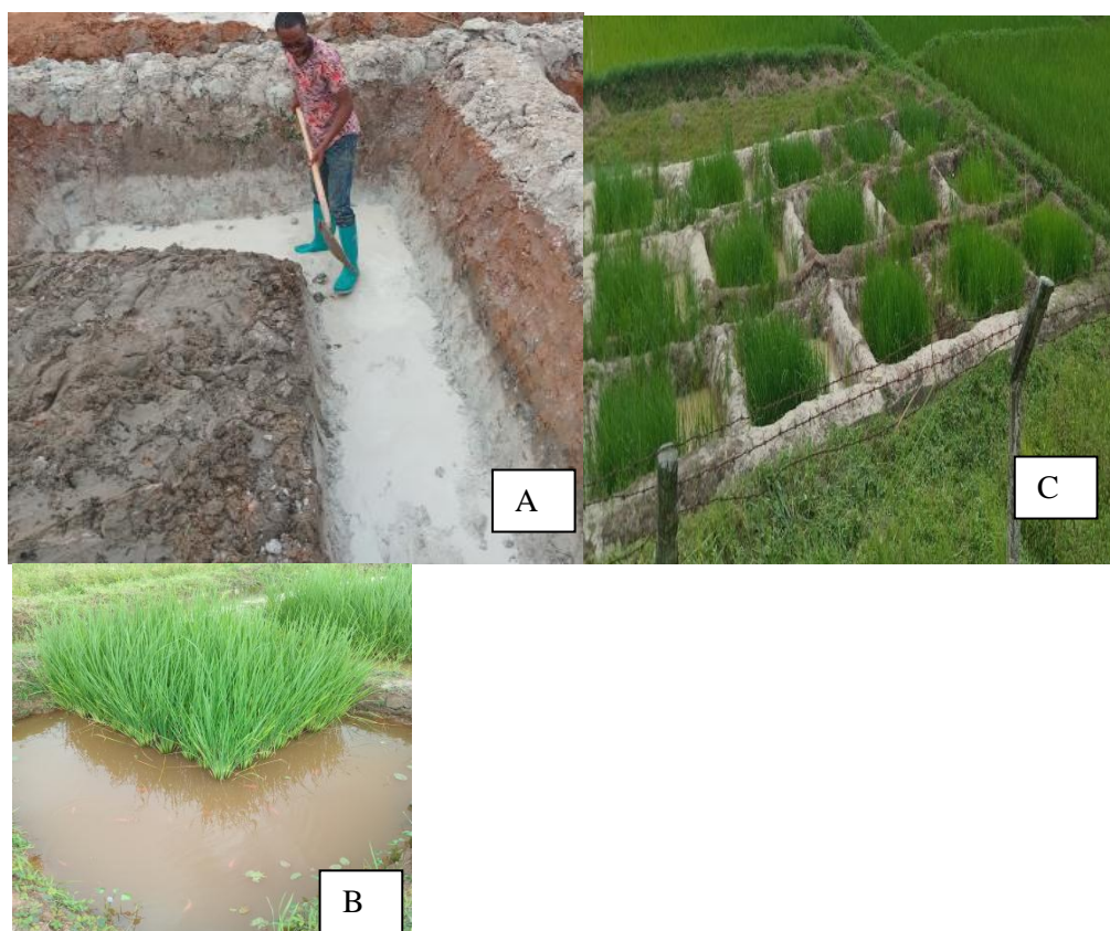
Figure 8: Field lay out (A) Pond construction diagram, (C), Research field diagram and (B) View of how each plot was designed
