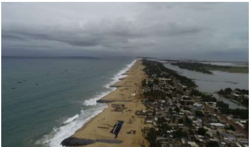
Figure 10: The groyne field at Blekusu captured using UAV in May 2022 (Charuka et al., 2023a)
