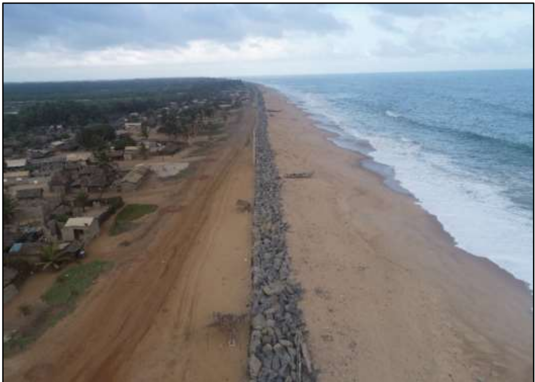
Figure 53: Atorkor revetment adjacent to the Anloga - Anyanui road
