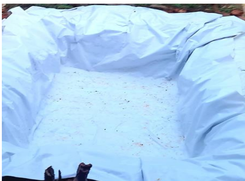
Figure 20: Tarpaulin Lining in the Constructor Fish Pond.
