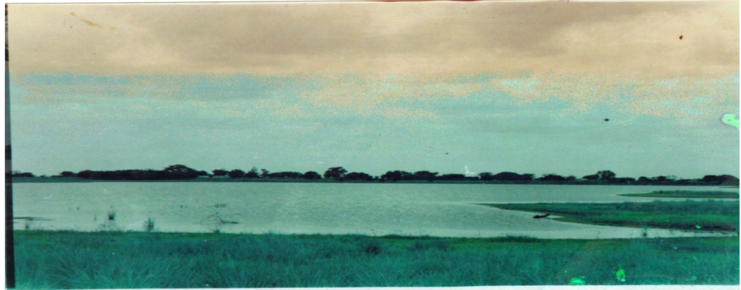
Plate 1: Wiaga irrigation dam
