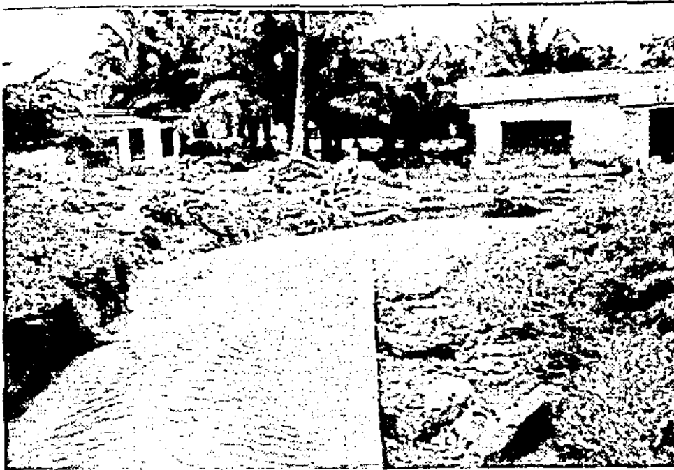
Plate 6: Diversion of a stream channel due to a building across the normal course of the stream, North Kaneshie
