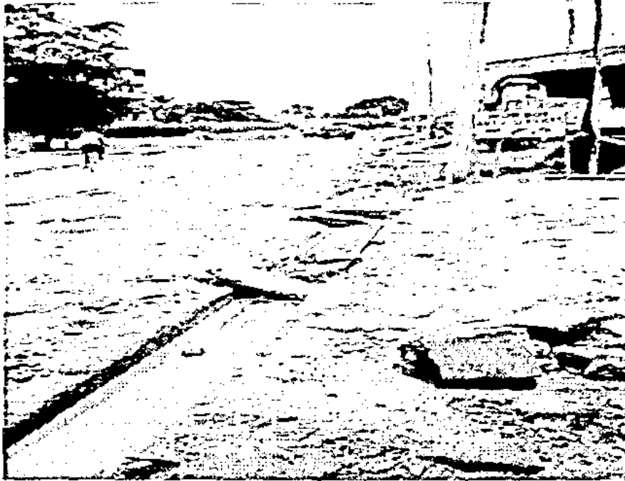
Plate 4: Drain filled with sediment, Swan lake
