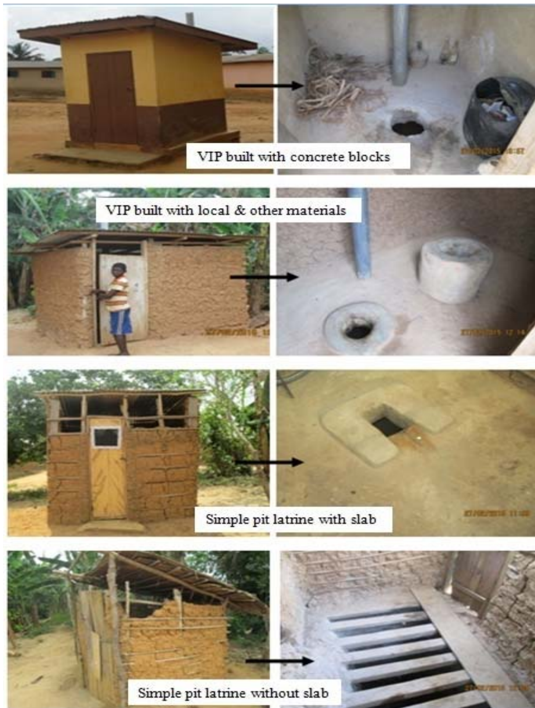
Plate 1: Type of household latrines constructed after CLTS intervention
