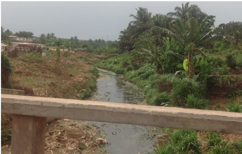
Plate 3: A choked channel at Bakado
