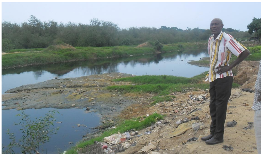
Plate 2: A choked drain at Adakope
