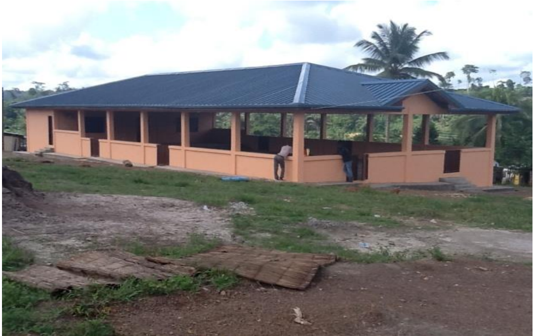
Figure 3: Subriso Community Centre
