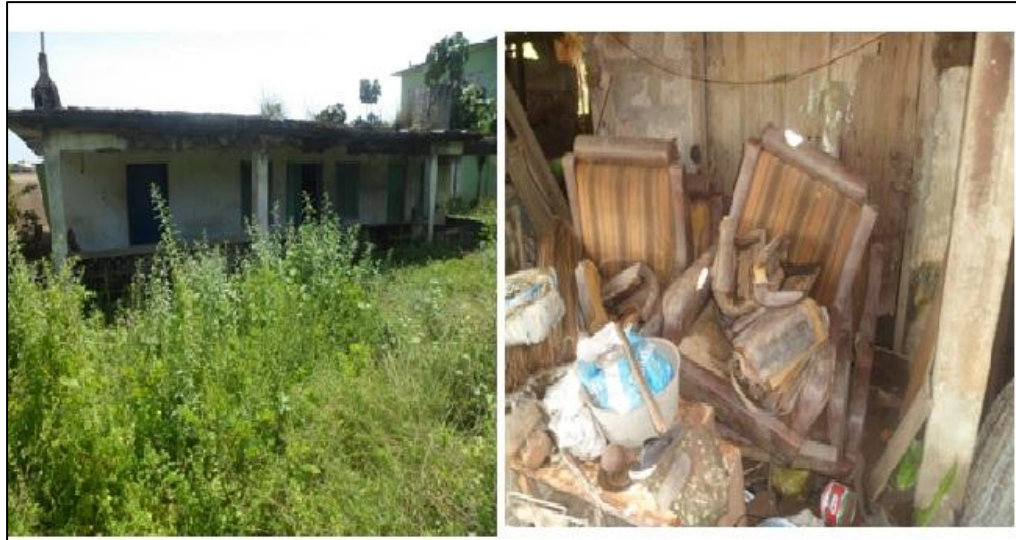
Plate 5: Abandoned house and furniture destroyed by flood
