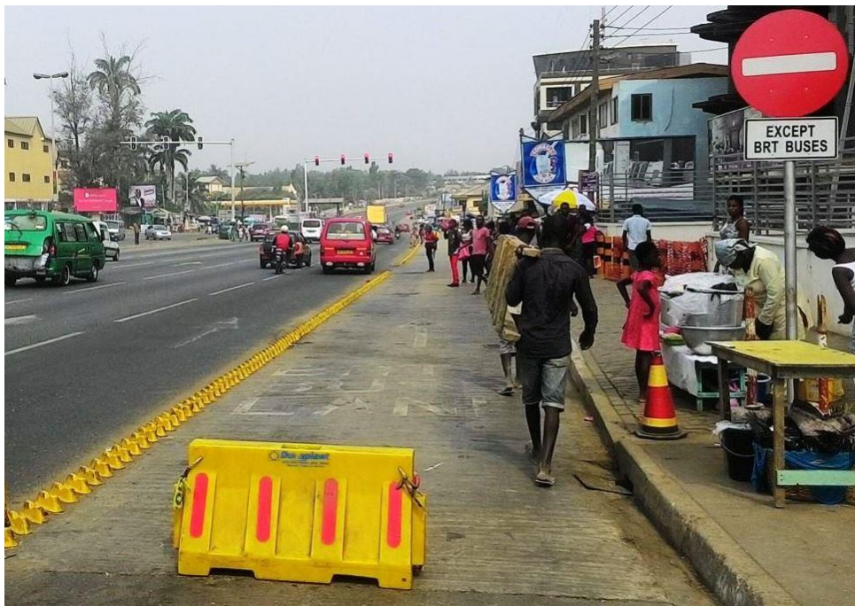
Figure 11: A Section of GAMA BRT Dedicated Lane
