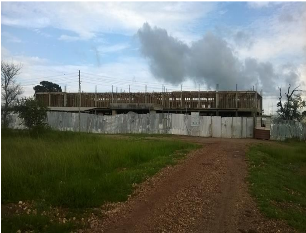
Figure 3: UCC CoDE Satellite campus under construction in Zuarungu, UE/R
