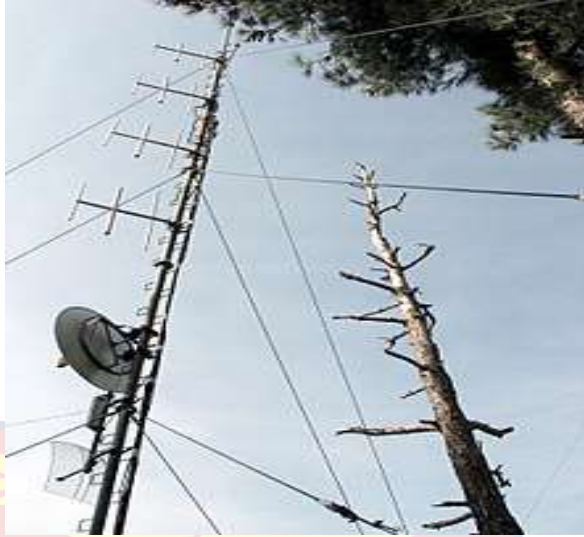
Figure 7: A photograph of a collinear antenna array
