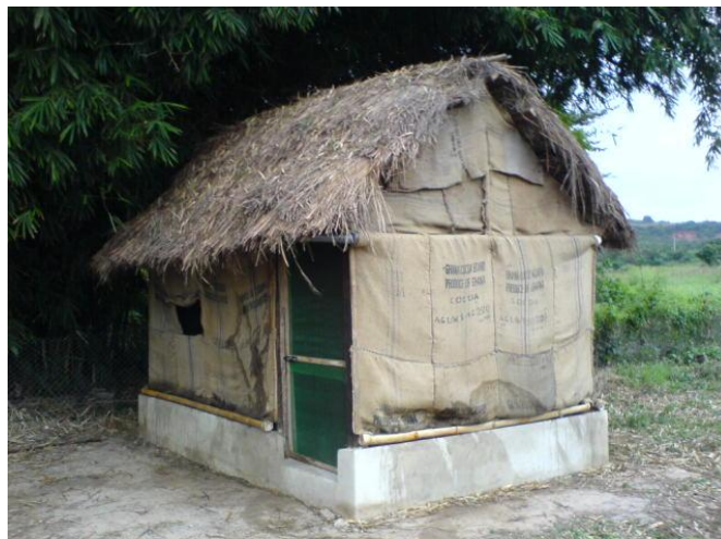
Plate 6. Evaporative cooling barn
