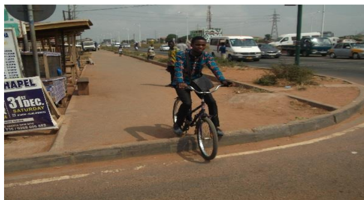
Figure 20: Dead-end of bicycle lane impeding free flow of riding
