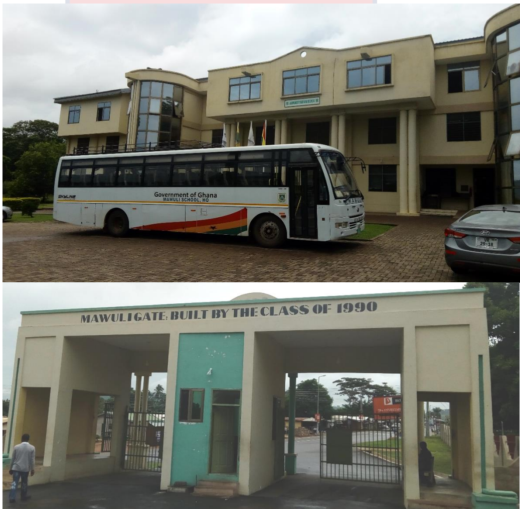
Figure 2: Forecourt & Main entrance of Mawuli School
