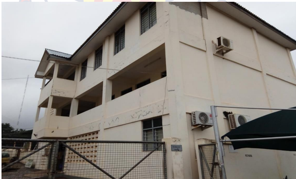
Figure 4: Administration Block of CMC of EPUC in Ho
