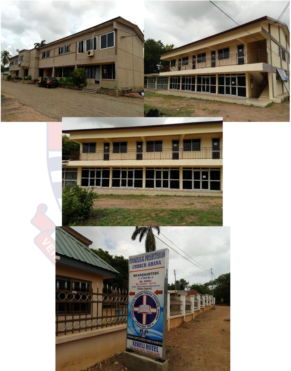
EPCG Headquarters in pictures
