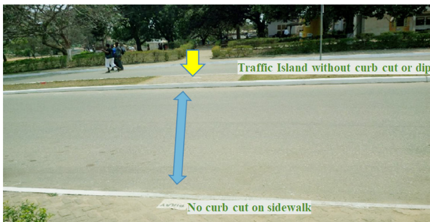
Plate 8: Traffic Island without zebra crossing and drop curbs when approaching the Science Faculty
