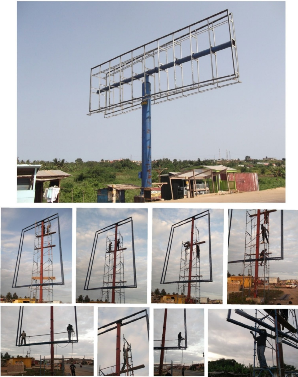
Figure 3. Installation of modern billboards. Source: Fieldwork, 2016.
