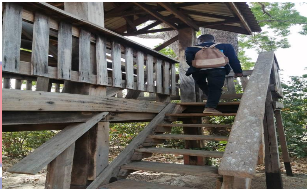
Figure 10: Watchout Tower at MNP
