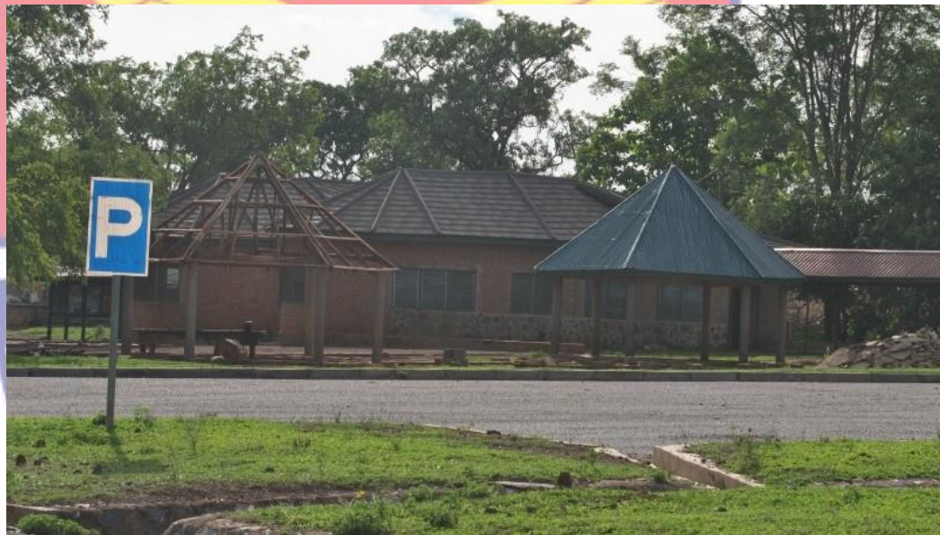
Figure 5: A Sign Post Showing Direction to Car Park at MNP
