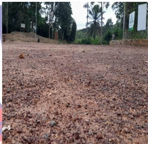
Figure 3: Car Park at KNP
