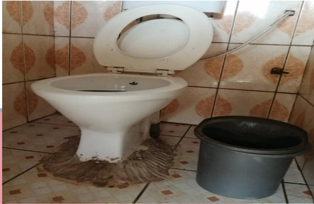
Figure 11: Toilet Facility at MNP
