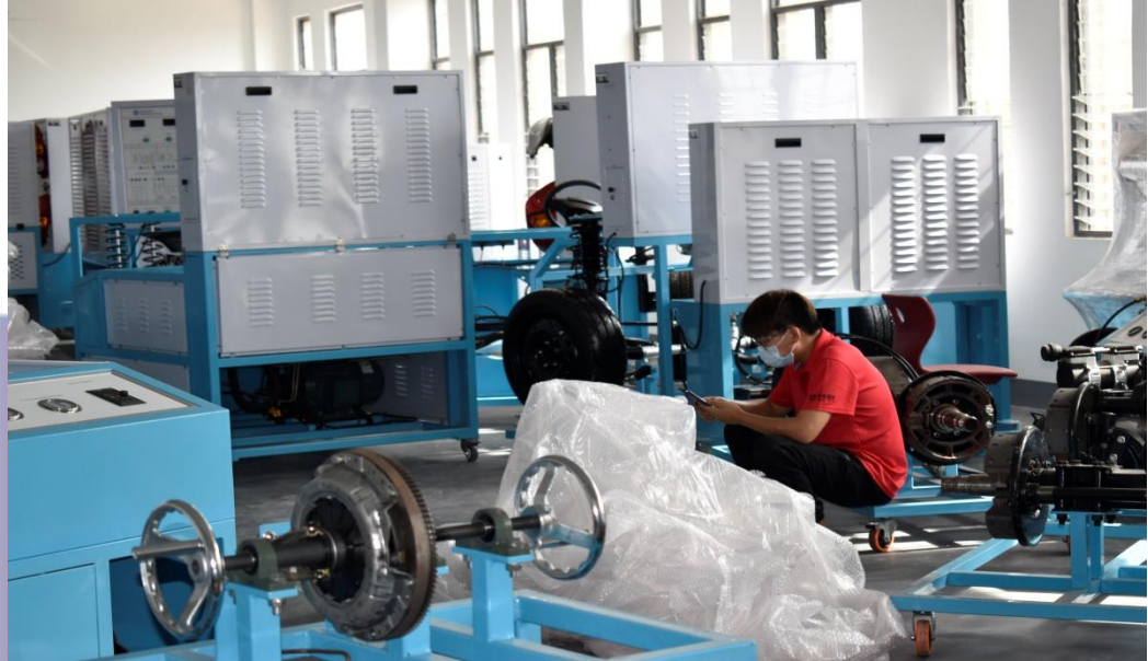
Plate 2: Chinese engineer installing AVIC laboratory and workshop equipment at Cape Coast Technical University.
