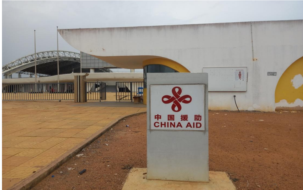
Plate 1: Front view of the Cape Coast Stadium built by the Chinese as part of its development aid programmes in Ghana.
