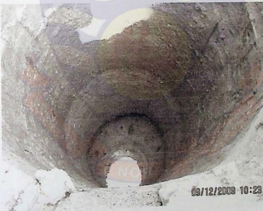
Figure 22: Photograph of the inside of a hand dug well in the dry season.
