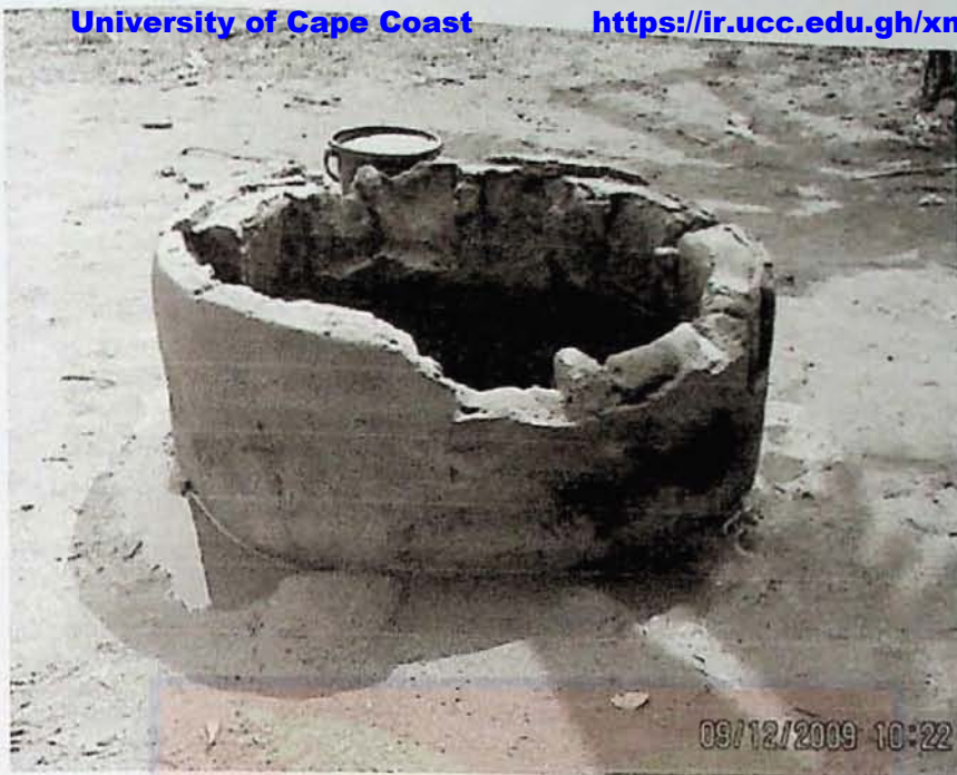
Figure 21: Photograph of the hand dug well at Kweikrom.
