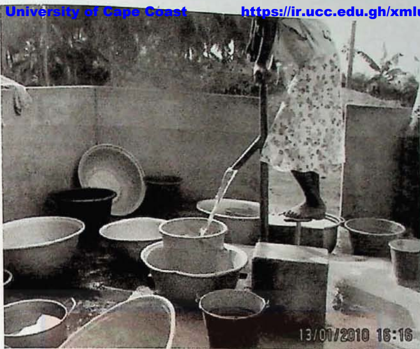
Figure 23: Photograph of a foot operated pump fitted to a Borehole.
