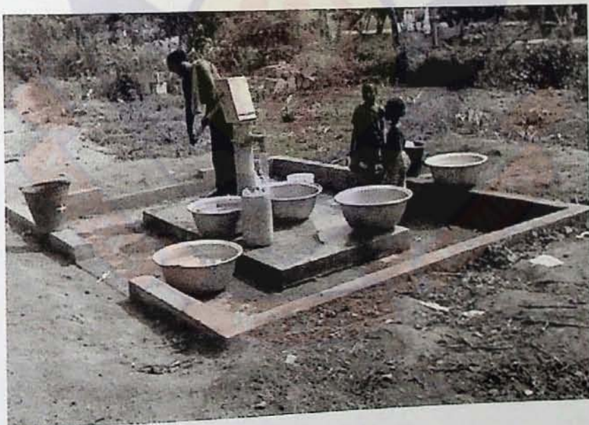
Figure 24: Photograph of a hand operated pump attached to a Borehole.
