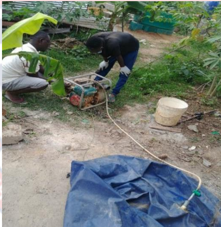
Figure 26: Biogas being utilized to power a generator
