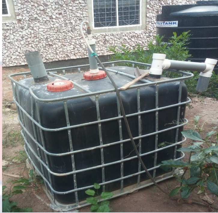
Figure 7: Portable continuous biogas plant
