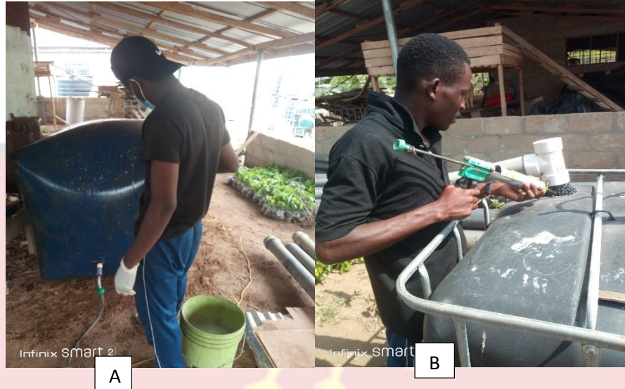
Figure 8: A= Checking for leakages on the balloon, B= Sealing of leakages on the reactor
