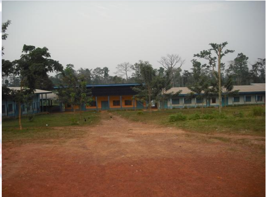
Plate 3: A school built by Newmont at Kenyasi new site
