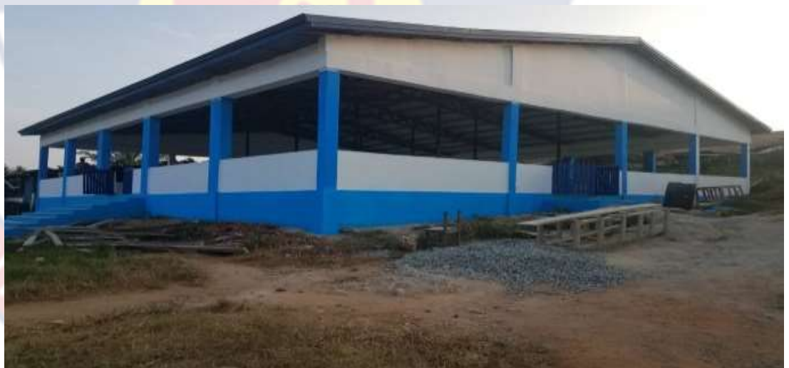
Figure 10: Dining Hall Facility for Assin Nyankumase Community Source: Fieldwork, Koufie (2021).
