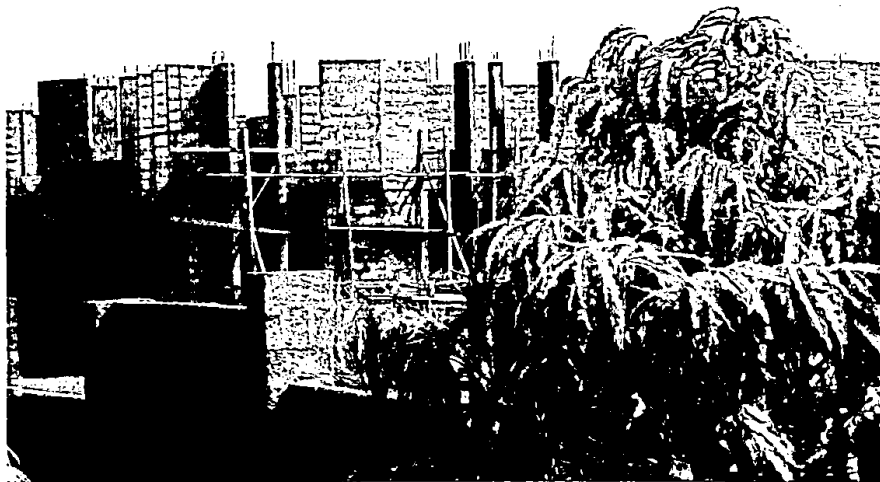
Plate 1: A Hotel Complex under Construction in Wa
