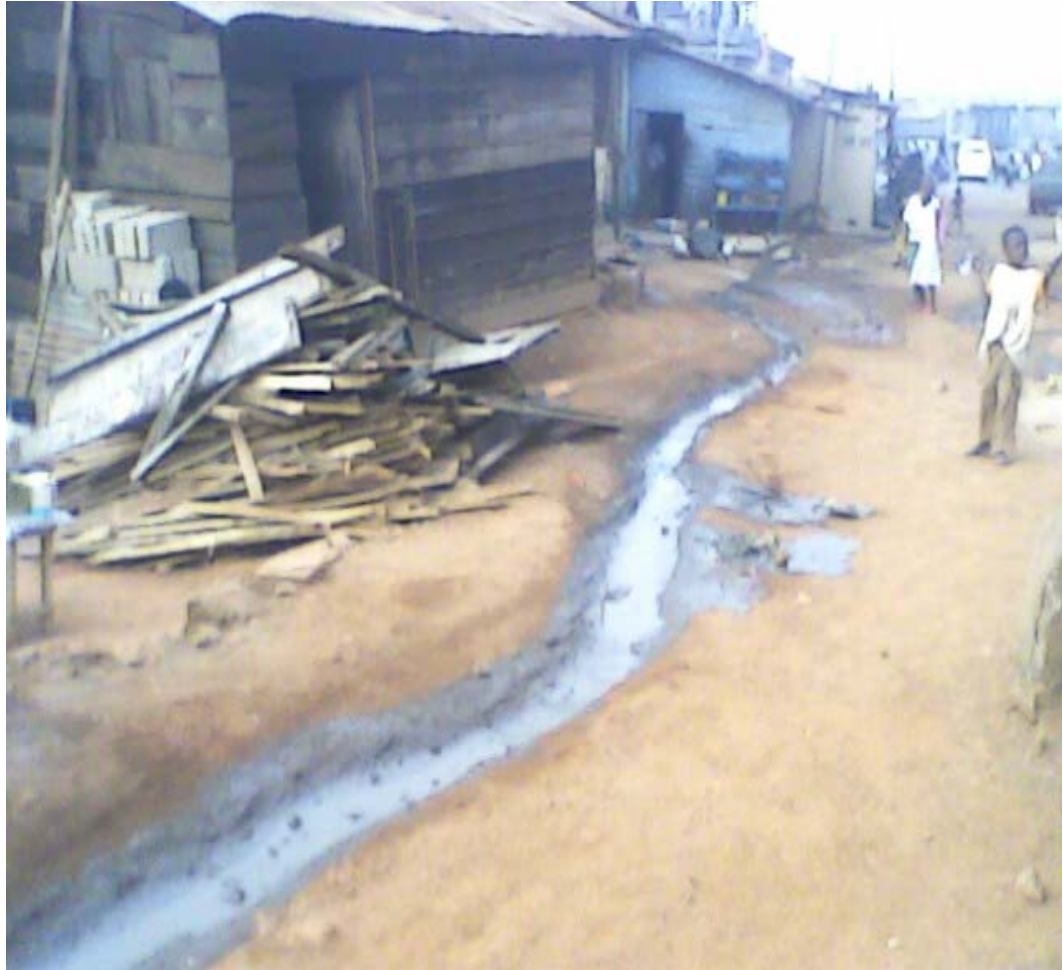
Plate 1: Evidence of unauthorised structures at Aboabo
