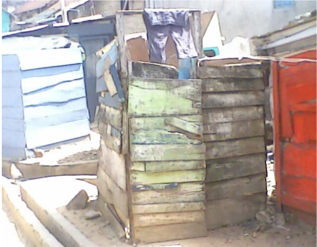
Plate 4: Bathroom structures at Aboabo
