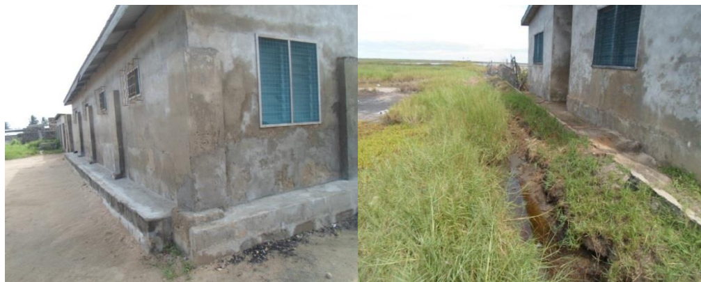
c. Built concrete around houses d. Temporary drainage
