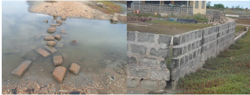
a. Temporary bridge b. Wall built around the houses
