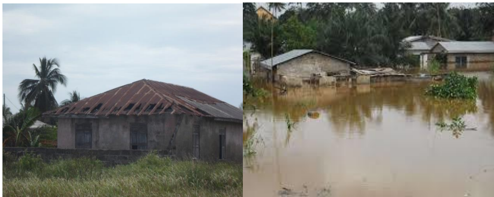
d. Abandoned completed buildings near the lagoon
