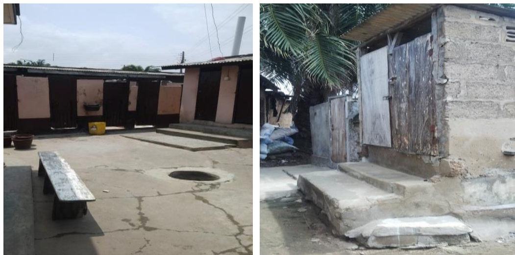
Figure 10: Bathroom and toilet facilities
