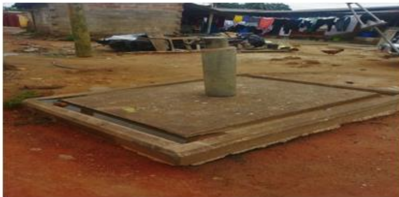
A Non-functioning Public Borehole in Doryumu
