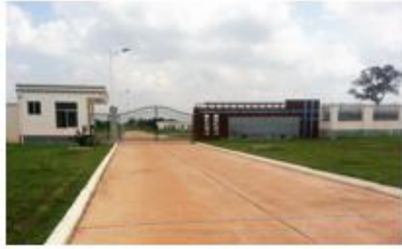
Entrance to water booster station in Dodowa
