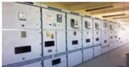
Monitoring station where flow monitored and controlled.
