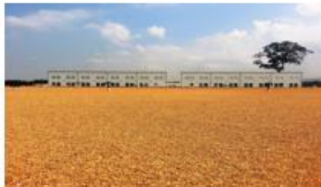
Top of the water storing tank
