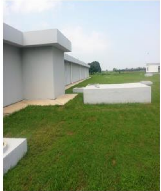
Side view of the storage tank
