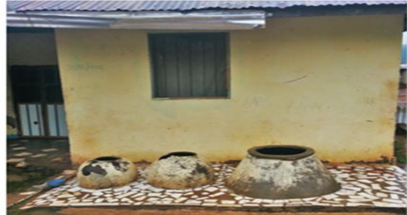
Clay and cement pots for harvesting and storing rainwater
