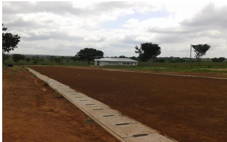
Plate 2. Bui CHPS Compound
