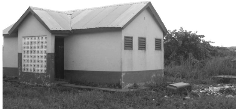
Plate 6. Washroom building in Basic School A
