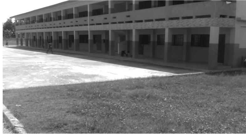
Plate 3. Front view of the JHS block of Basic School B
