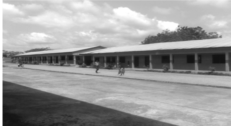
Plate 16. Primary classroom block in Basic School B
