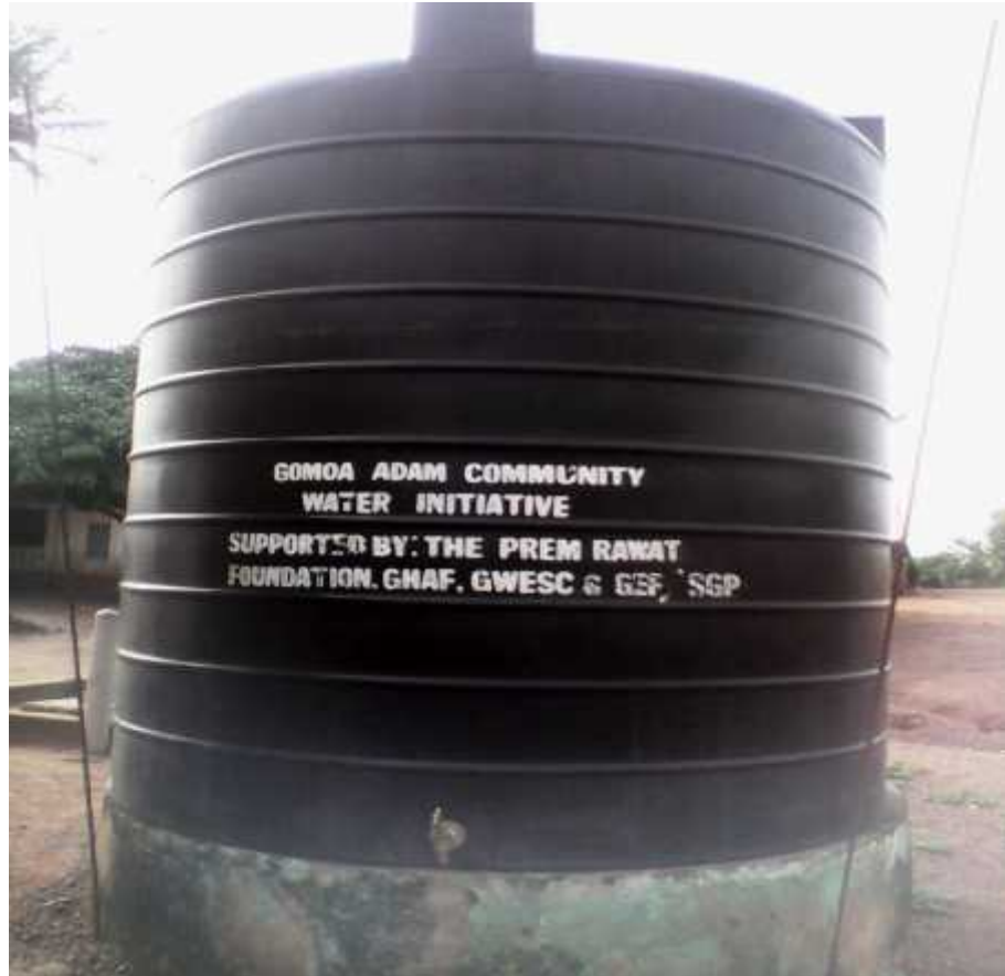
Plate 7: Poly-tank provided for Water Storage at Gomoa Adam
