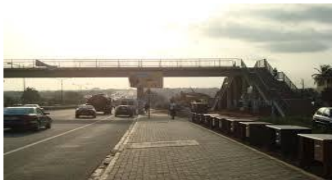
Unsuitable highway overpass for physically challenged and visually impaired
