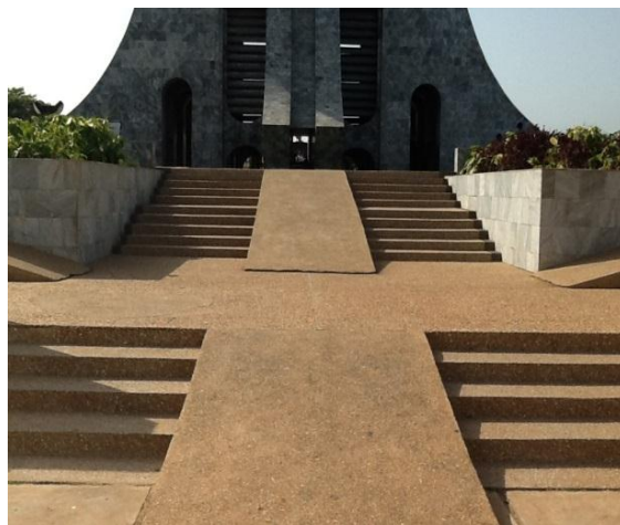
Suitable ramps for physically challenged
