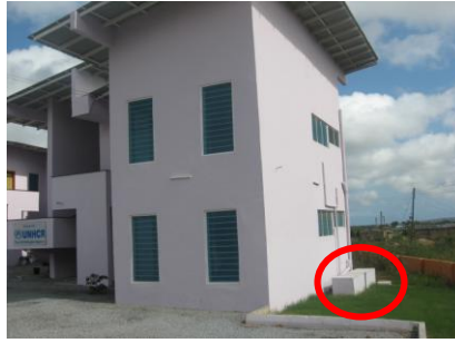
Figure 3: A biofil digester installed in a household (Photograph by Biofil)
