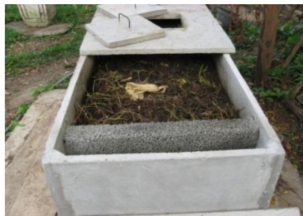
Figure 1: An exposed biofil digester to show the solids where living organisms are meant to feed and digest the solid matter (Photograph by Biofil).
