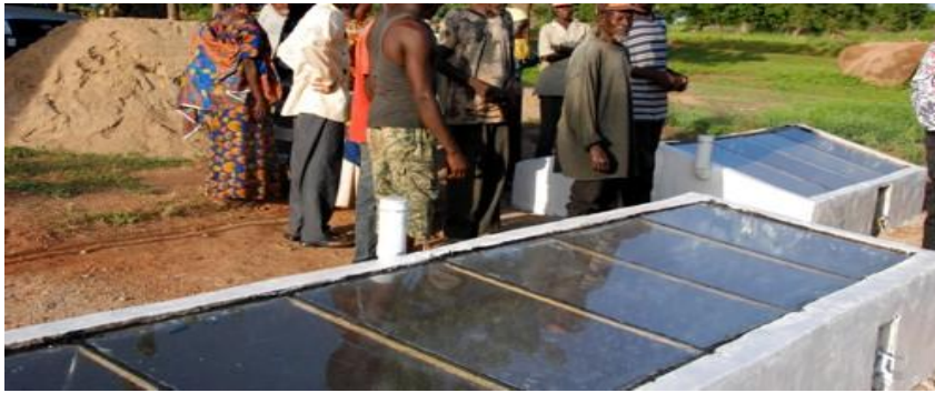
Figure 3: Solar stills constructed at Anafo Biisi Primary School in Bongo
