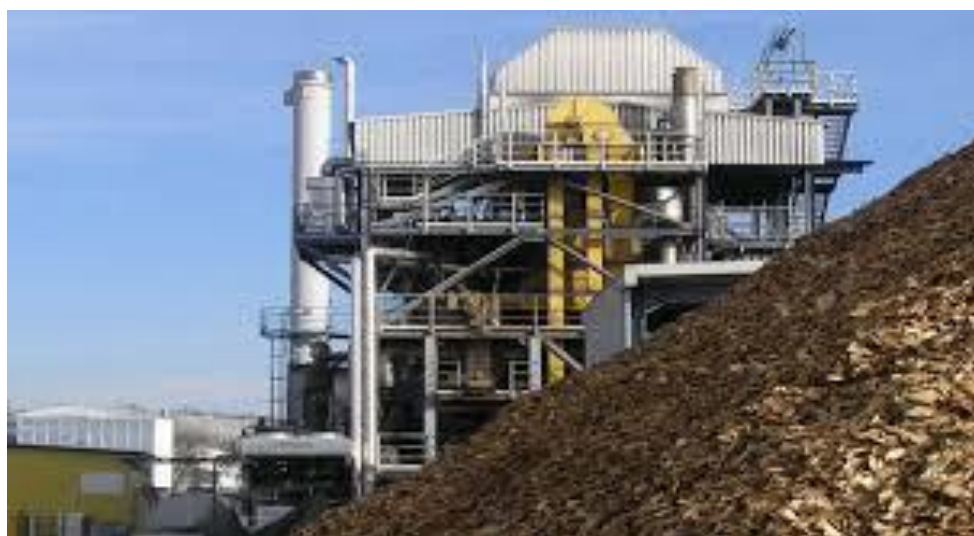
Figure 7: Overview of the Sludge Biomass to Electricity
