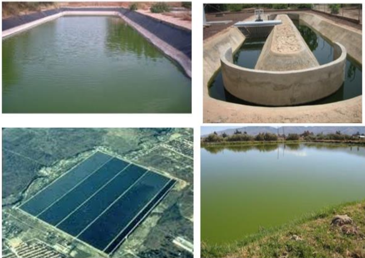
Figure 8: Overview of the stabilization pond with primary treatment and multiple facultative pond
